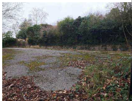
Photograph 4: Hardstanding and H1 to rear of B1
