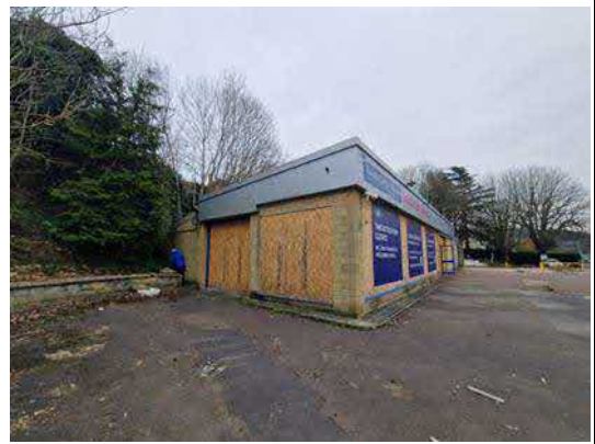
Photograph 2: Side elevation of B1
