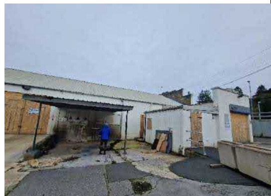
Photograph 6: Side elevation of B2
