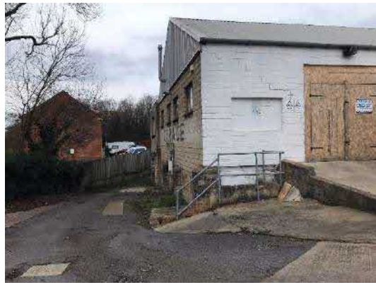
Photograph 7: Rear elevation of B2
