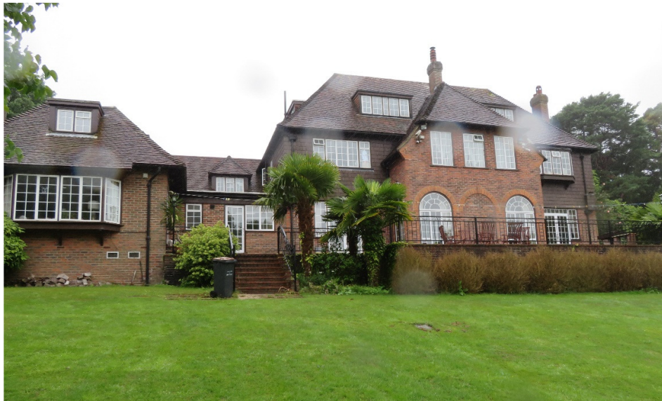
Photo viewing Rear of Property from Back Garden (Camera Facing South)
