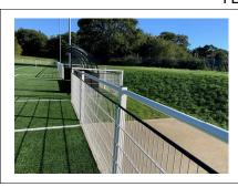
Zaun Spectator fencing with DUO8 (200x50) or Dura lock 3 rail fencing with mesh infill.
