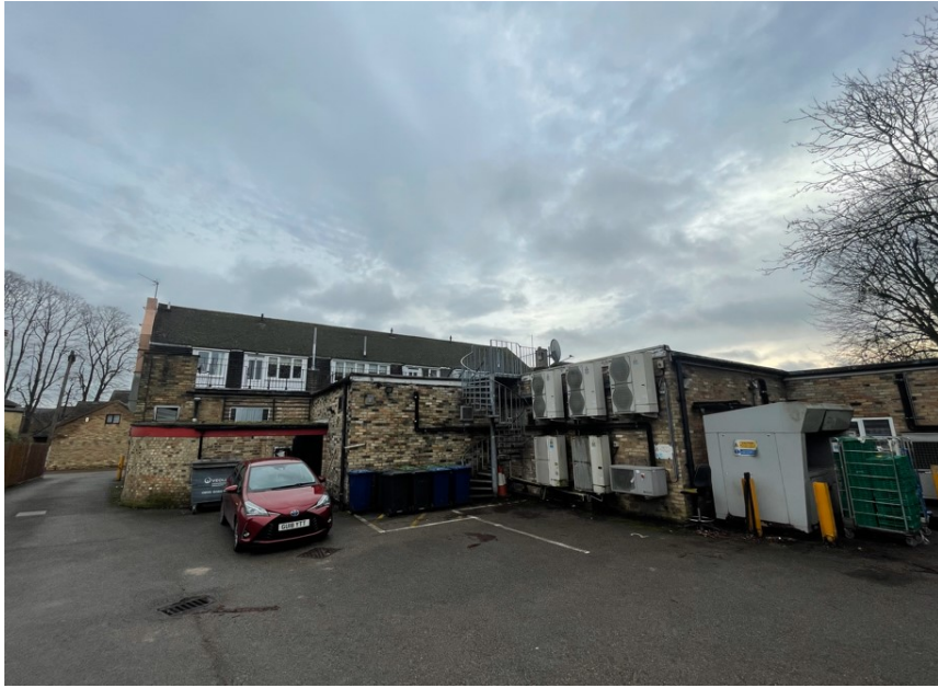
View of Rear Elevation
