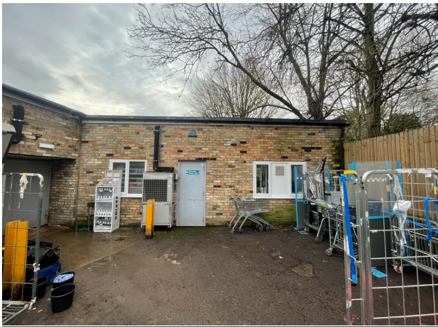
View of Rear Elevation
