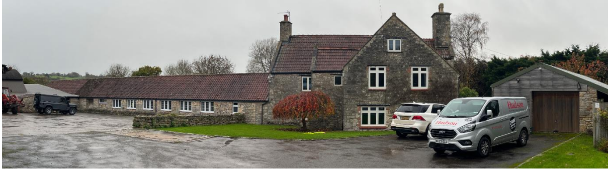
Figure 2 - East elevation of the farmhouse at Manor Farm.
