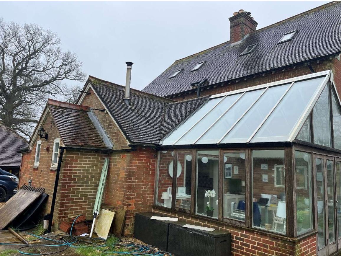
Figure 3. Northern and western elevations looking southeast.
