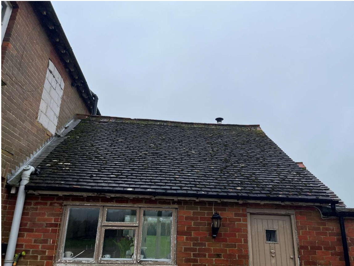
Figure 4. Eastern face of northern elevation looking west.
