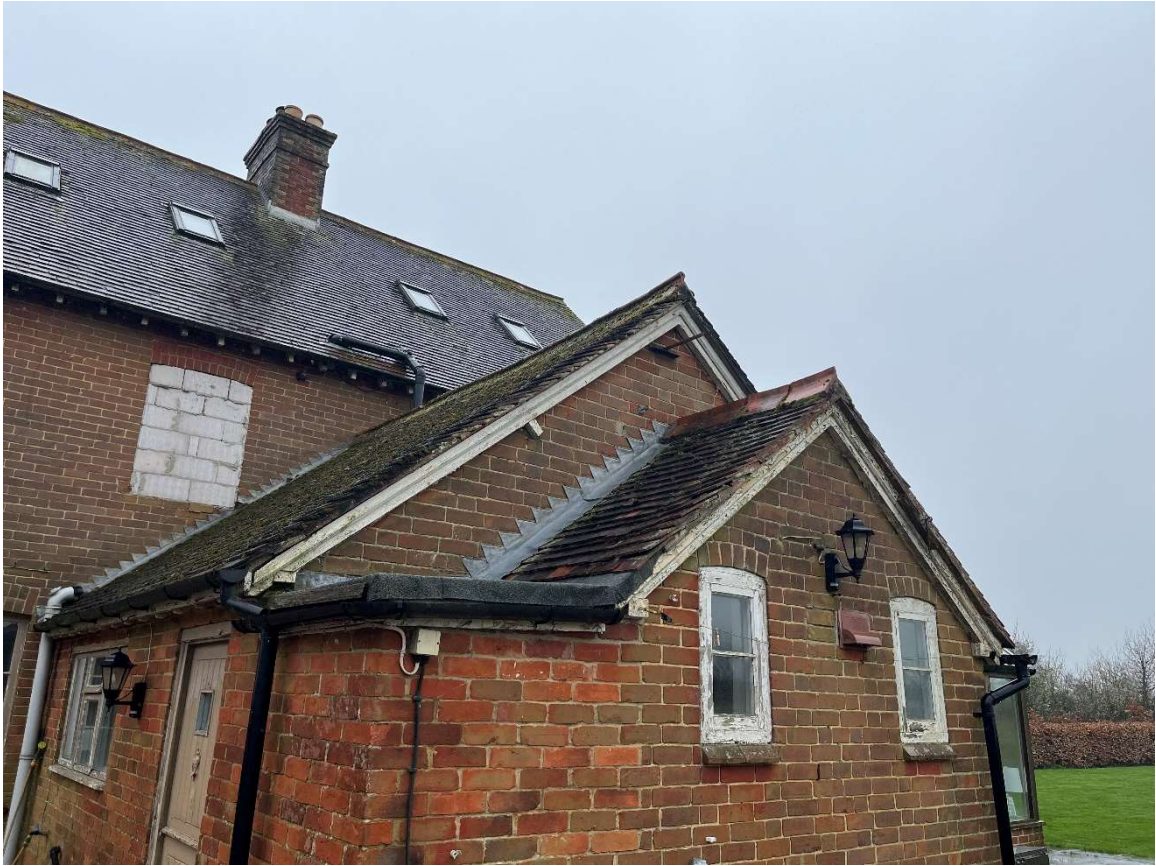
Figure 2. Northern elevations looking southwest.
