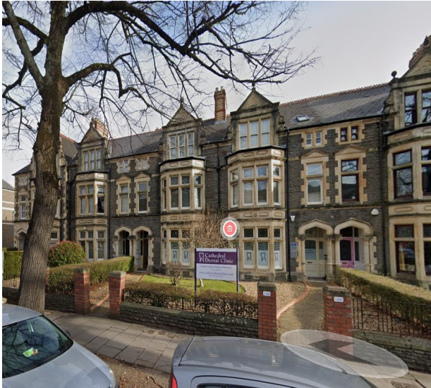
Front elevation of application property
