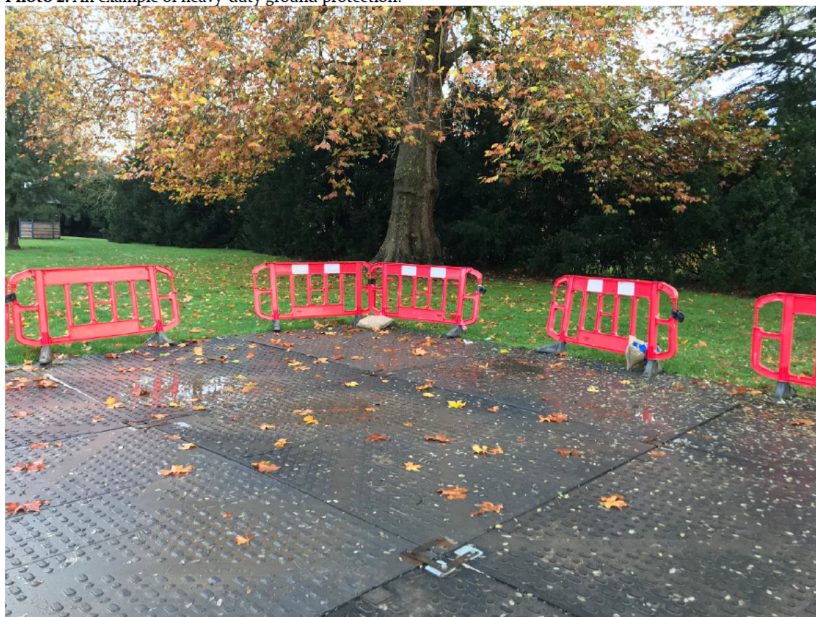
Photo 2. An example of heavy-duty ground protection.
