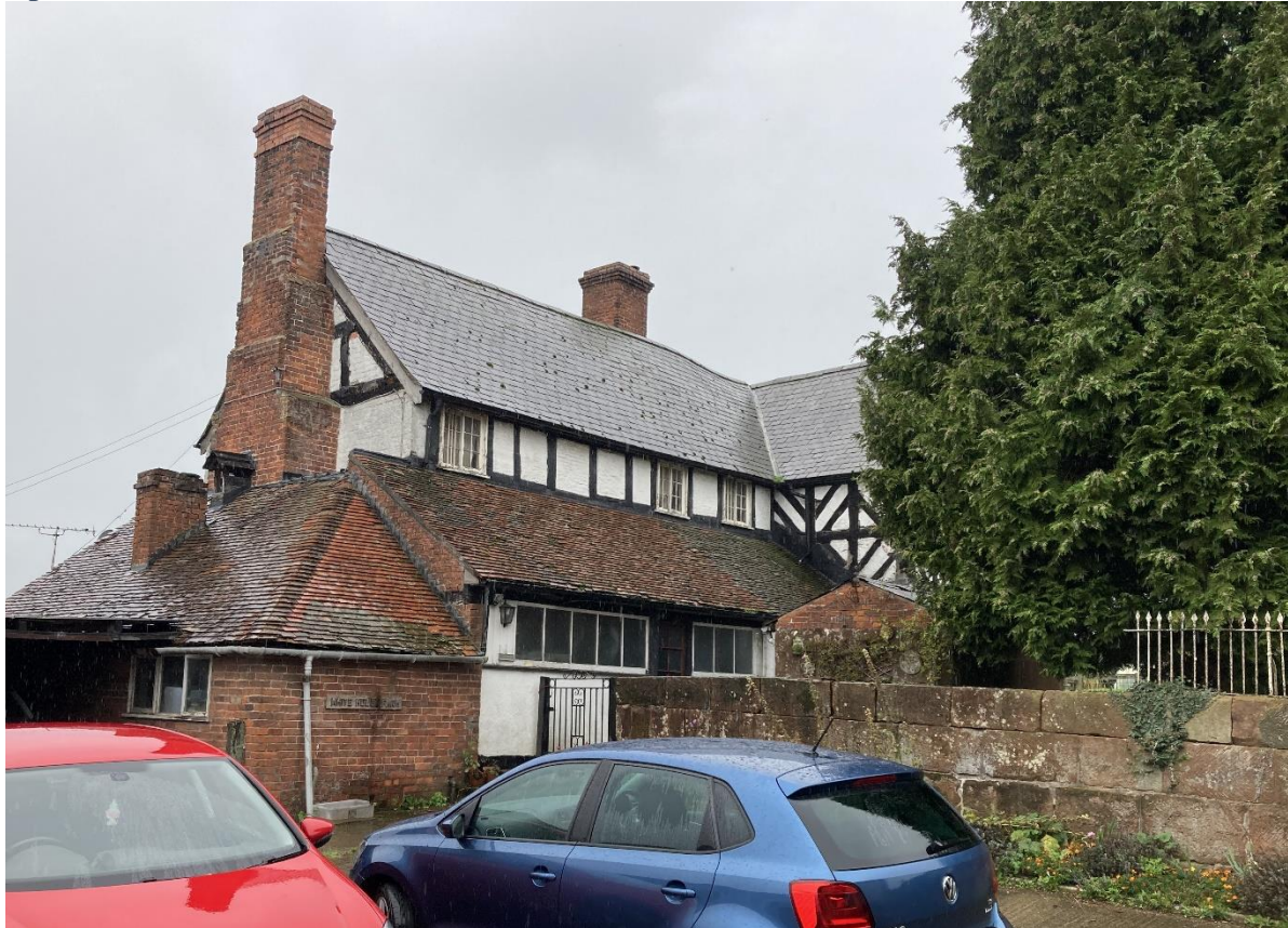
Figure 8: North Elevation of White House Farmhouse
