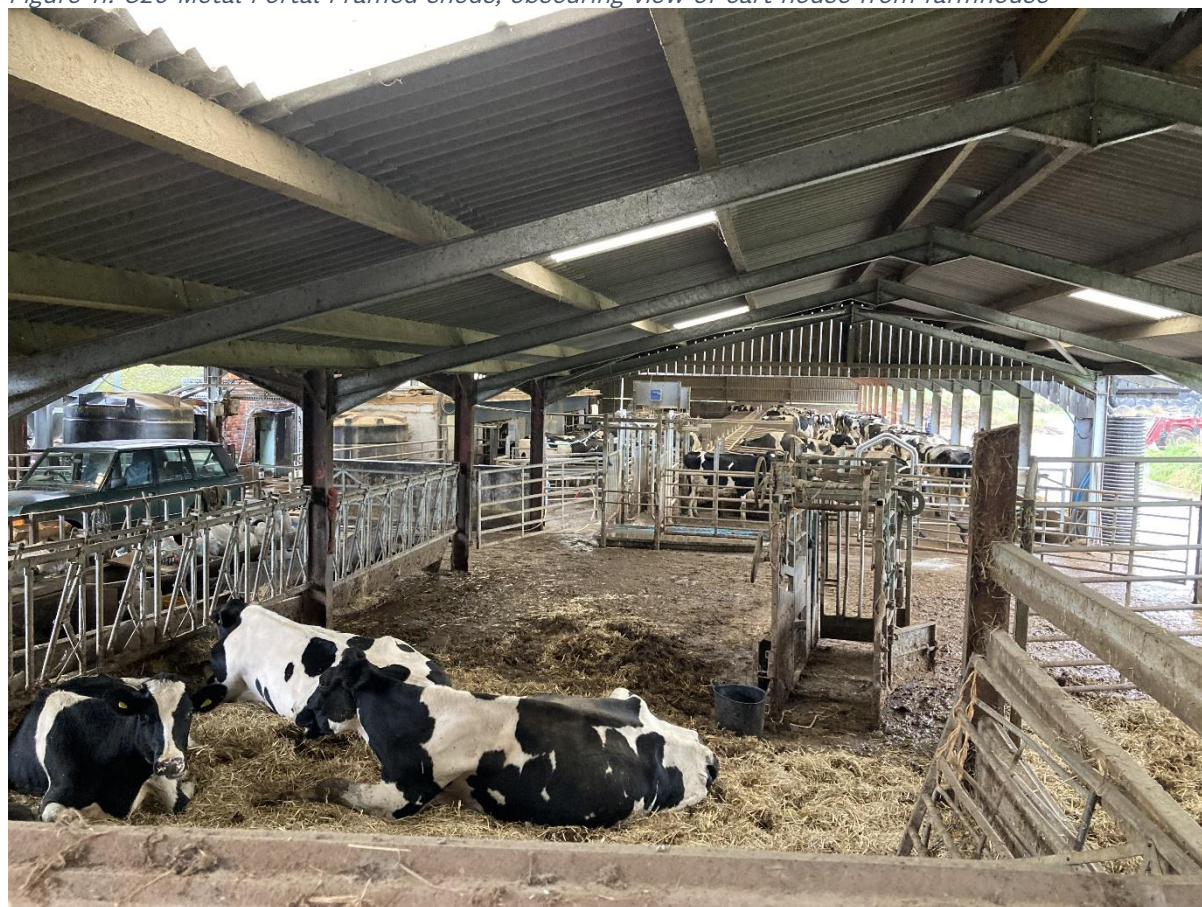
Figure 11: C20 Metal Portal Framed sheds, obscuring view of cart house from farmhouse
