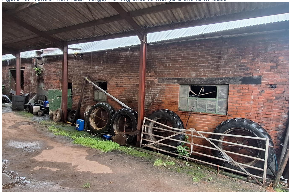
Figure 10: Front of north barn range, fronting onto former yard and farmhouse
