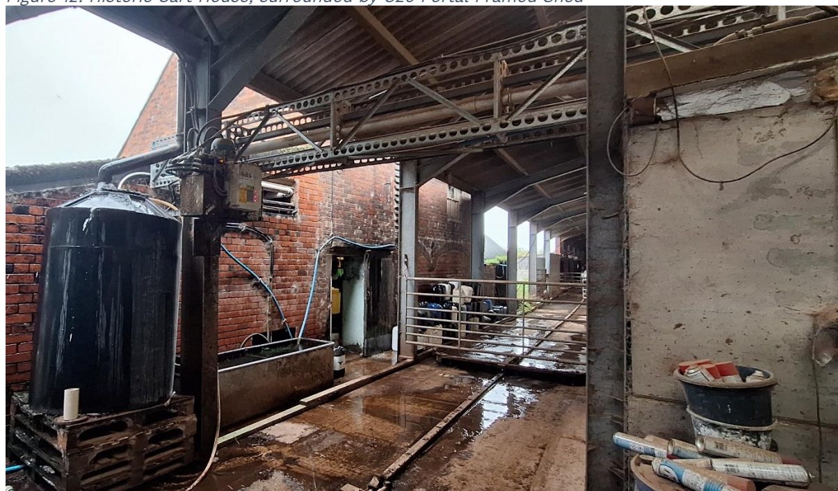
Figure 12: Historic Cart House, surrounded by C20 Portal Framed Shed
