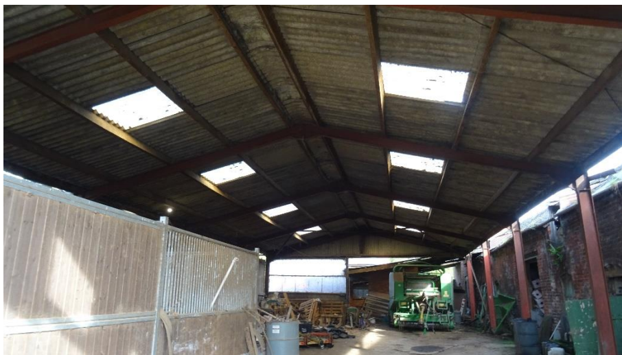
Figure 3. Inside material/equipment storage area
