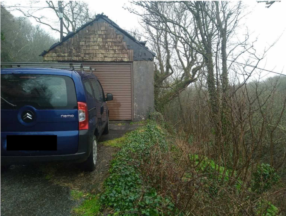
Photo 1: garage south-eastern aspect
