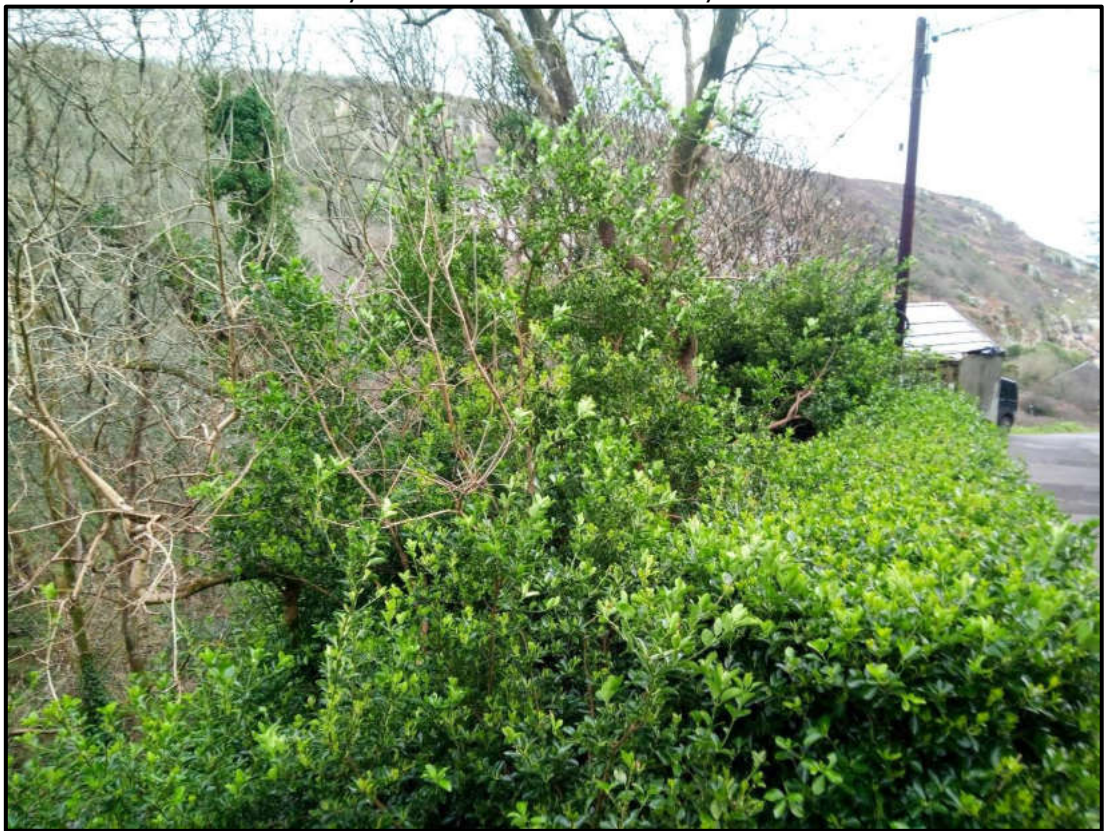
Photograph 4: View from the northwest corner of the property looking southeast towards the garage and shed.
