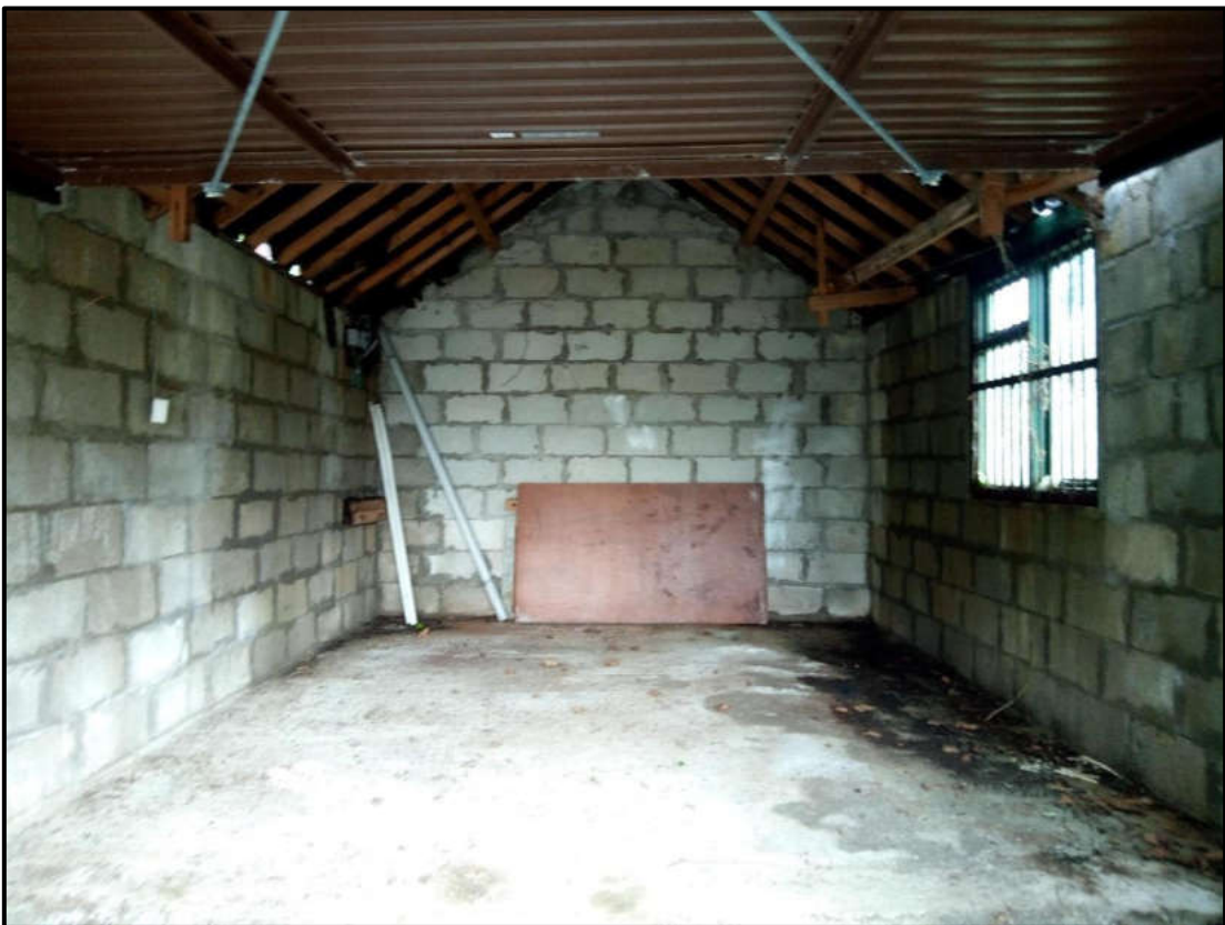
Photograph 8: View looking northeast inside the garage.
