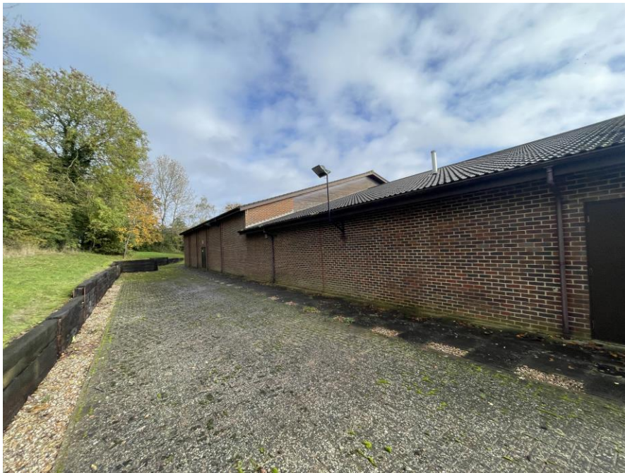
Figure 6 – View facing the side of the property.
