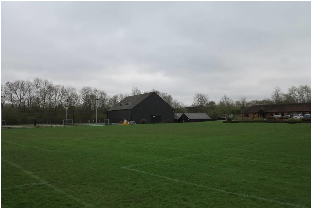
Plate 1. The sports hall and attached changing rooms seen from the playing field; the area of field in the foreground forms part of the Manor of the More scheduled monument
