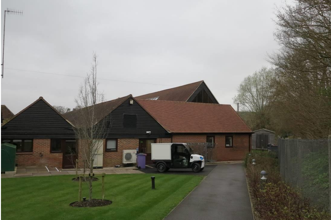
Plate 19. The school buildings from the east; the gable to the left relates to the listed stock shed (encased in later brickwork etc) while everything to the right of this is late 20 th - and early 21 st -century construction. The roof of the sports hall can just be seen in a filtered form directly above the garden shed on the right side of the image
