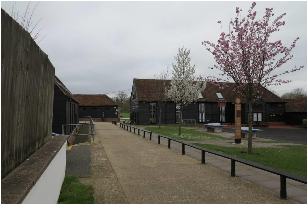
Plate 2. Converted threshing barn (right) on the western side of the former farmstead yard (the northern end of the listed calf shed outside the yard can be seen to the left)
