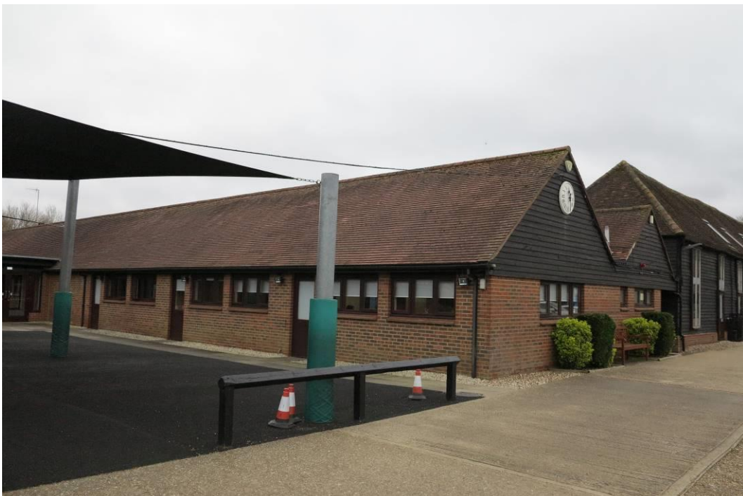
Plate 10. Modern school buildings to the north of the listed group (the gable to the right of this image relates to the listed stock shed, with the listed threshing barn to the right of this)
