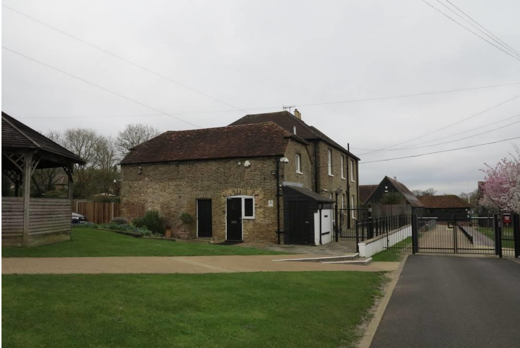
Plate 7. The former farmhouse seen from the entrance to the playground/former farmstead yard to the east
