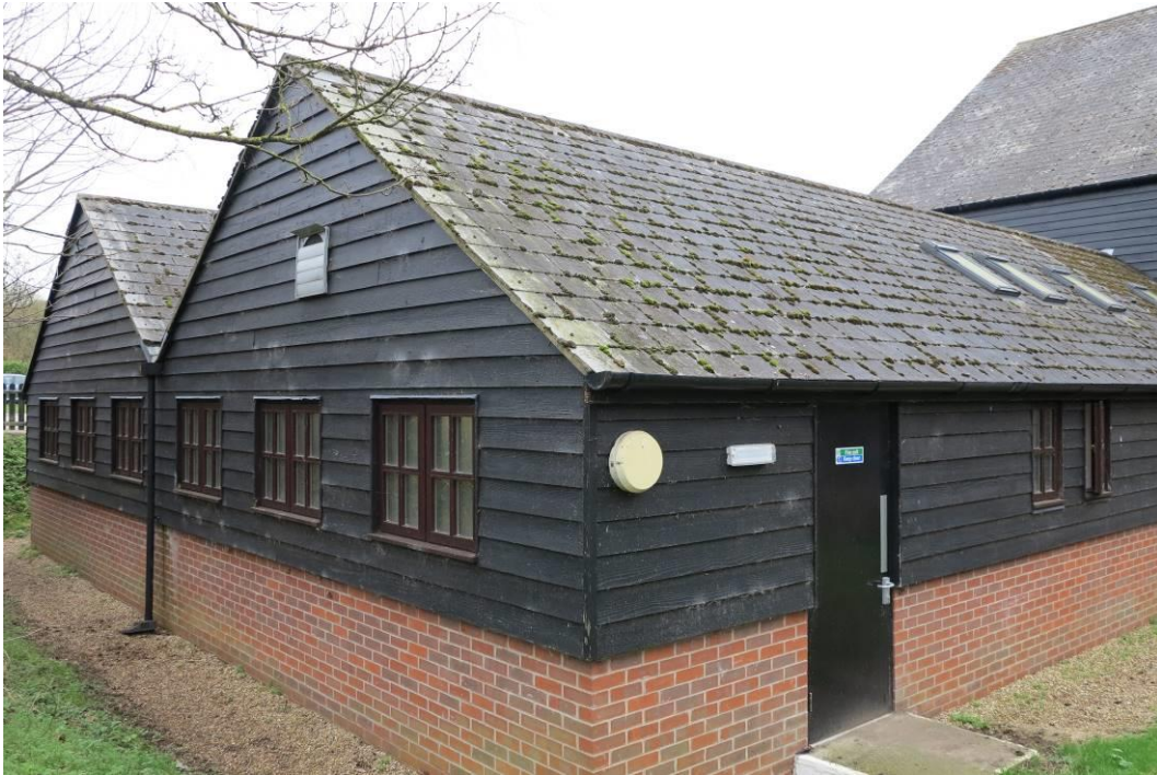
Plate 17. The changing rooms
