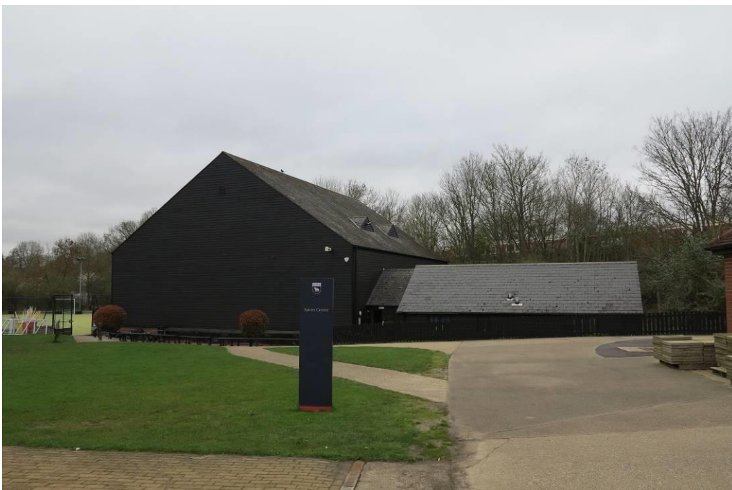
Plate 14. The sports hall and attached changing rooms
