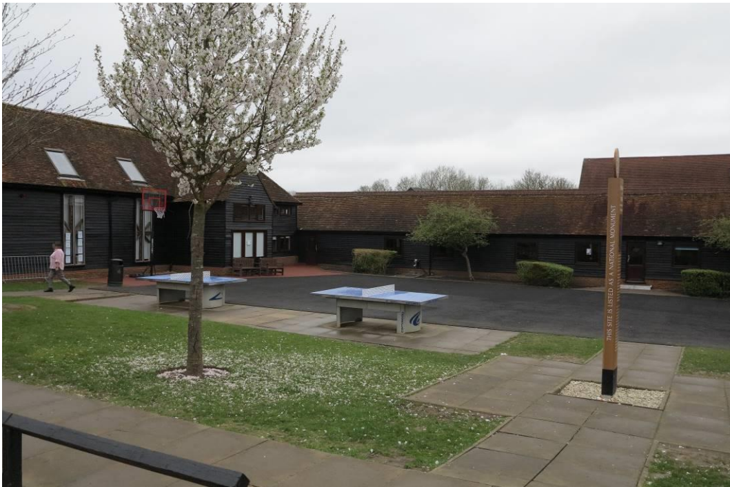
Plate 20. View northwards from the raised area at the southern end of the former farmstead yard (now a playground); the ridge of the sports hall can just be glimpsed towards the centre of the image above the listed former stock shed
