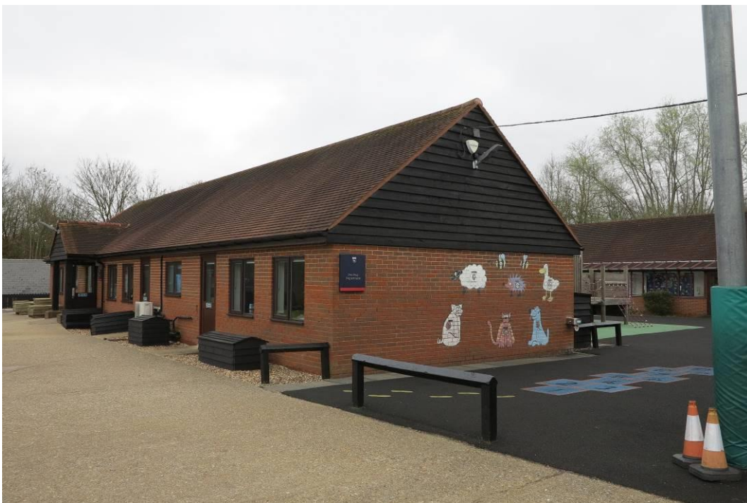
Plate 12. Modern school buildings to the north of the listed group
