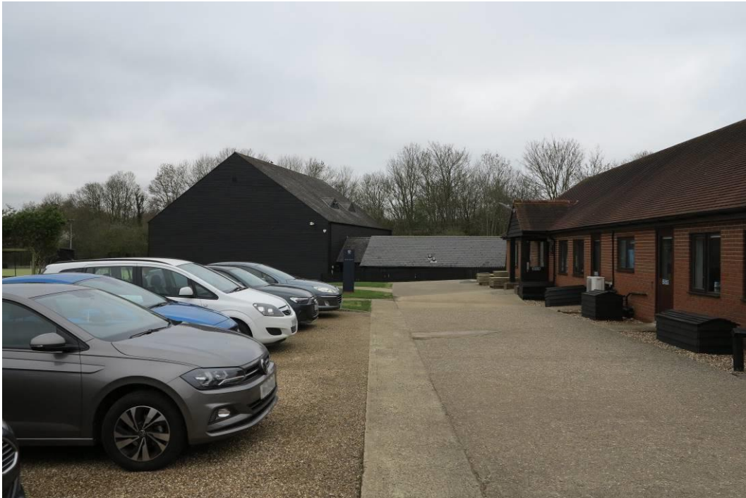
Plate 13. Modern school buildings to the north of the listed group, with the sports hall and attached changing rooms to the left
