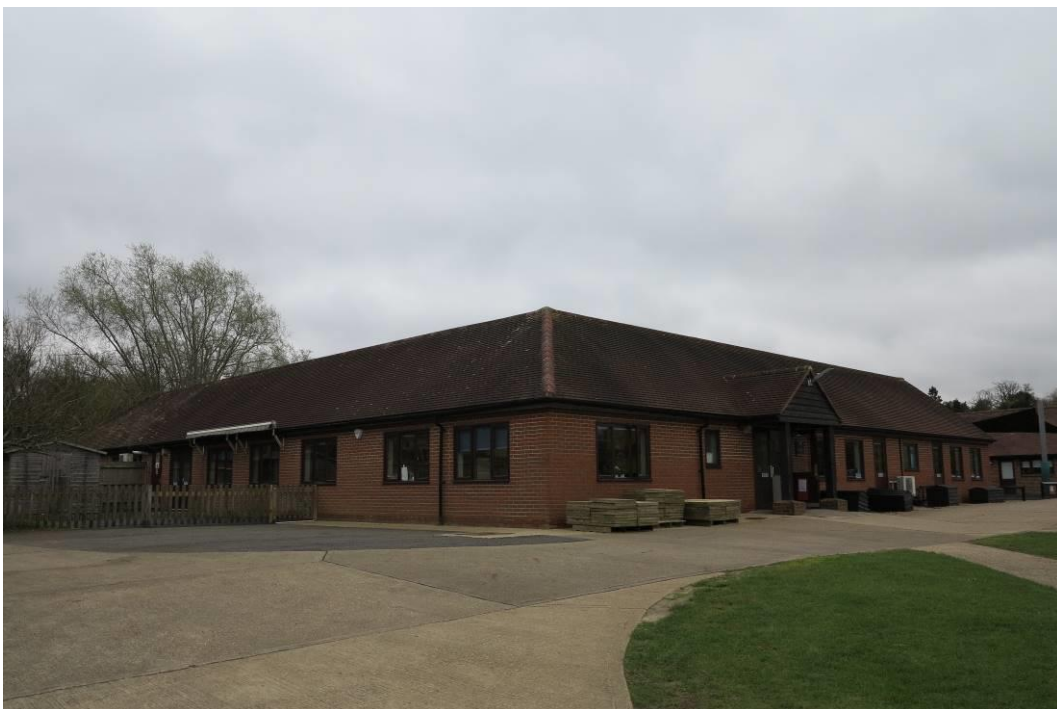
Plate 18. Modern school buildings located between the sports hall and the group of listed buildings to the south
