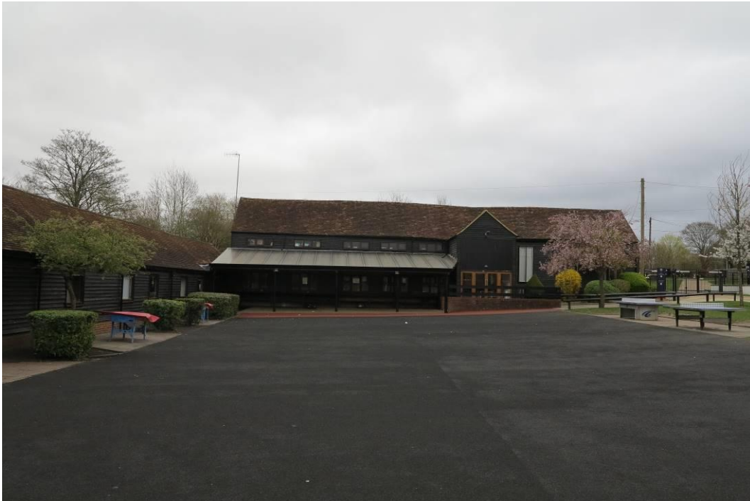
Plate 3. Converted barn on the eastern side of the former farmstead yard
