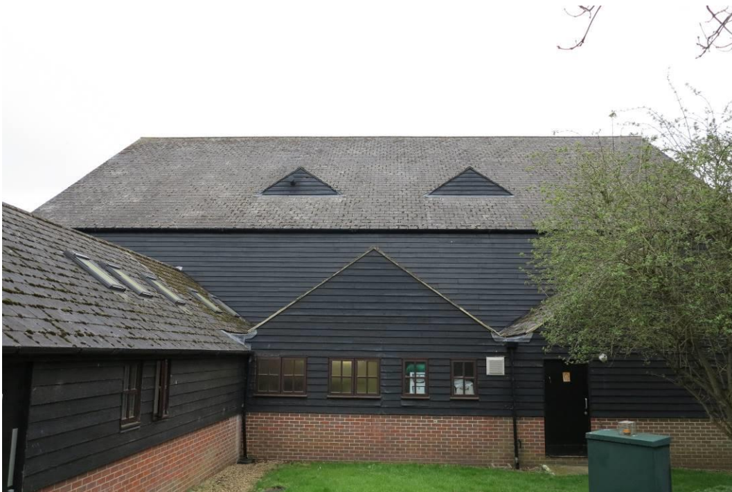
Plate 16. The sports hall and changing rooms from the east
