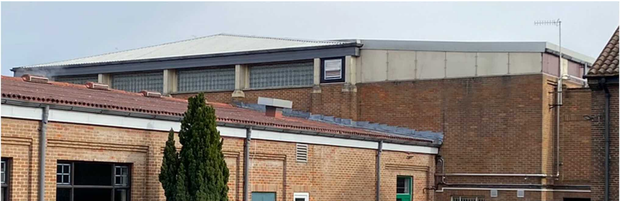
Photograph 1 – External view MTS Sports Hall.
