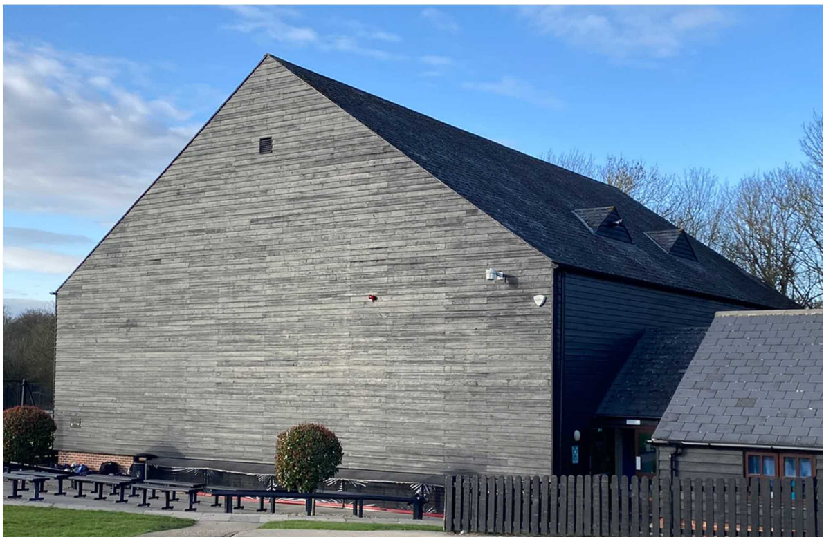
Photograph 6 – external view of MTPS Sports hall.
