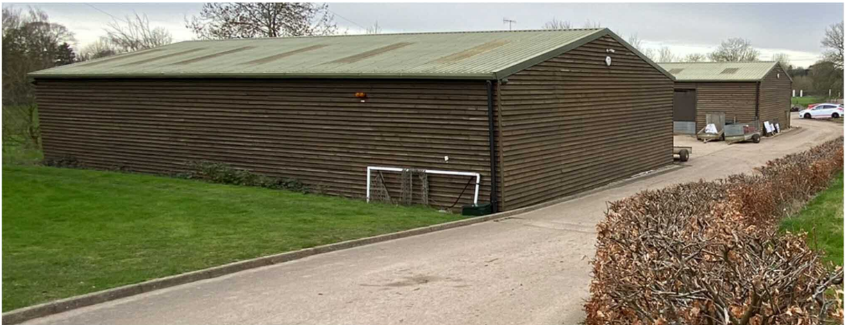
Photograph 4 – external view of MTS Grounds Maintenance building.
