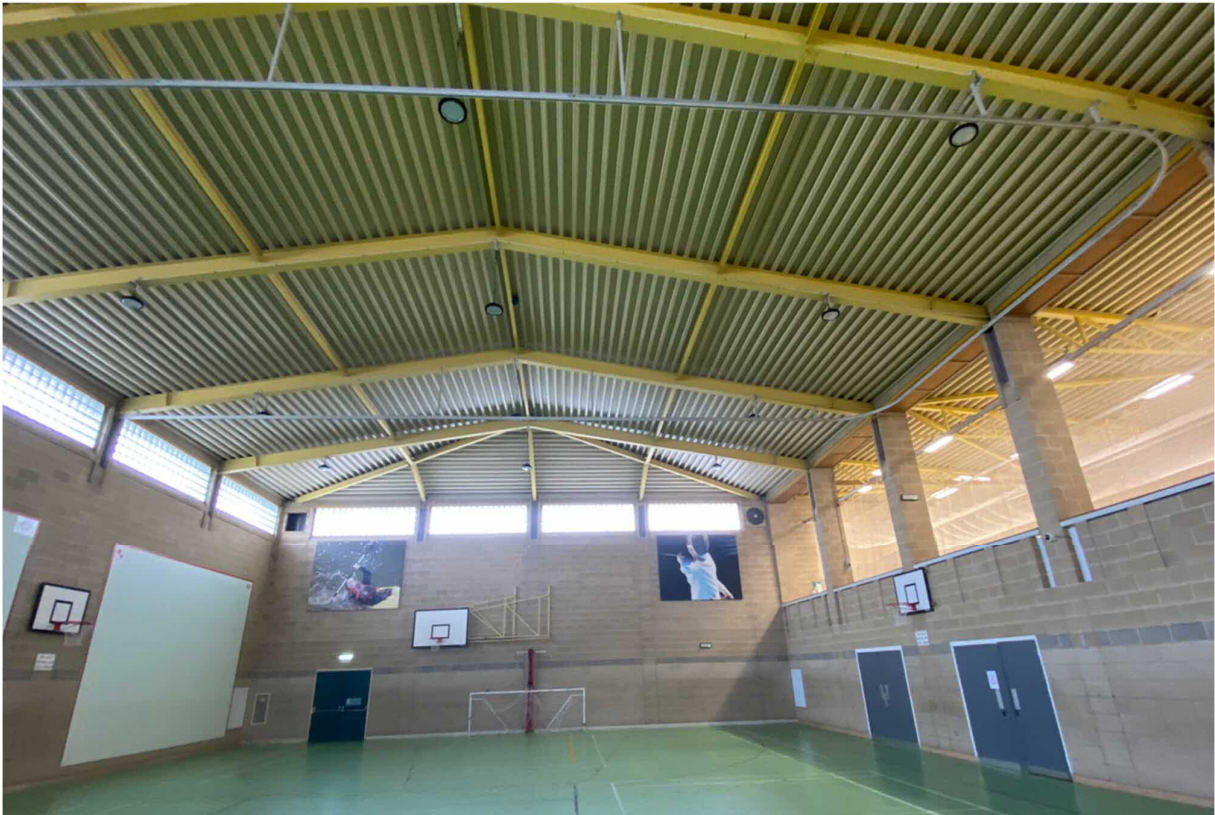
Photograph 2 – internal view MTS Sports Hall (main hall area).
