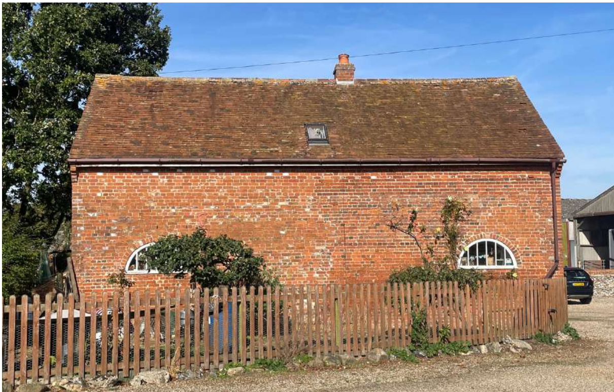
Image of existing property
