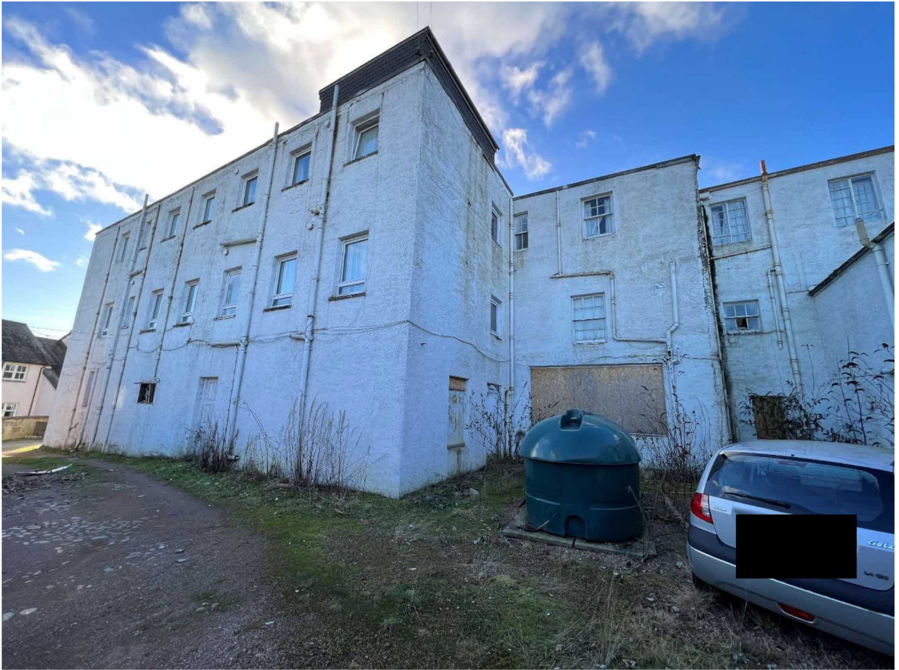
Photo 31 : Photograph of internal rear elevation of rear bedroom block to internal service area showing the array of window designs. A mixture of white timber sash and case, white timber casement, white steel casement and white pvc.
