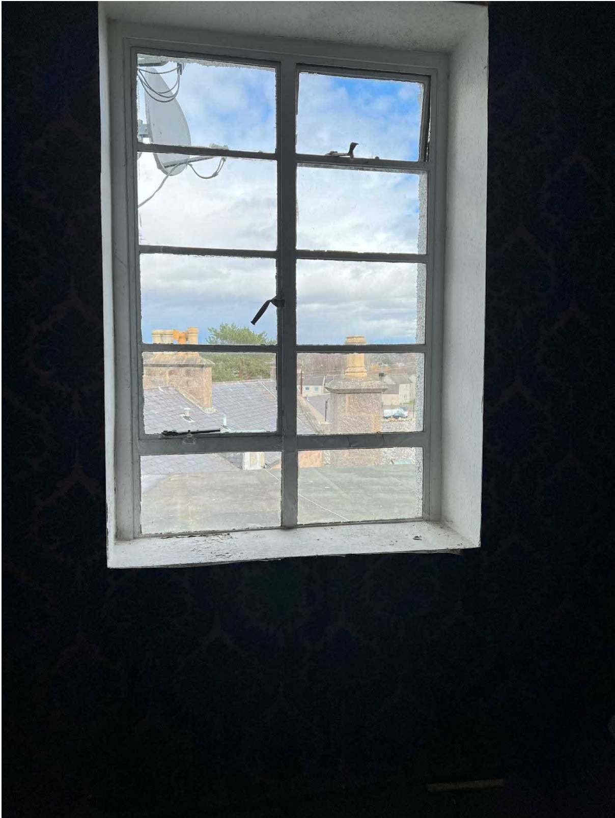
Photo 4 : Example of single glazed steel window to rear of the building.
